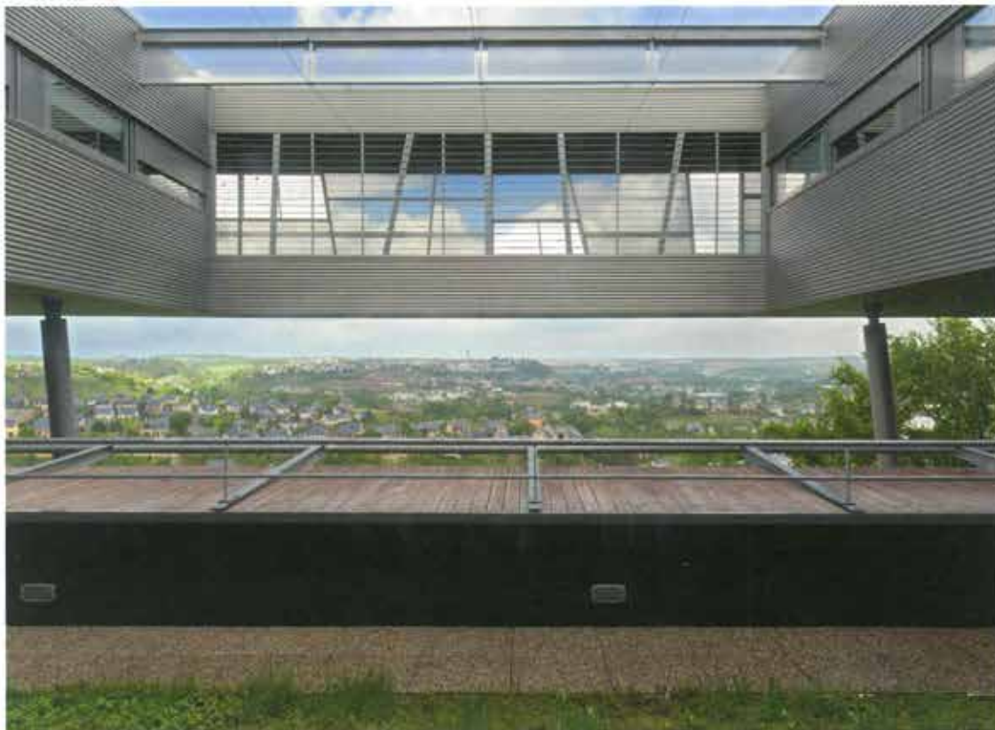
↑ Suspended walkways link the open ends of the H-shaped plan, creating two suspended 'air-patios'.
